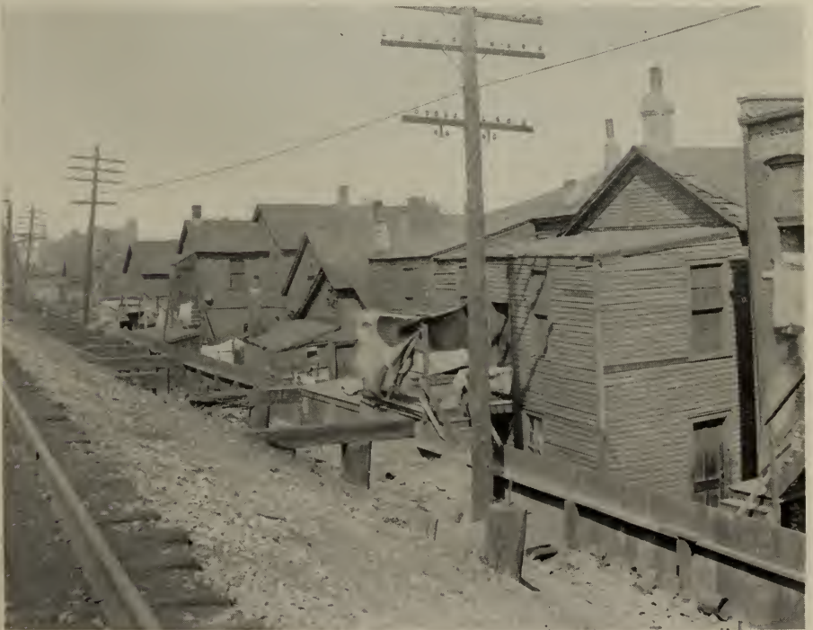
REAR VIEW OF HOUSES OCCUPIED BY NEGROES ON FEDERAL STREET Classified in text as "Type D"
